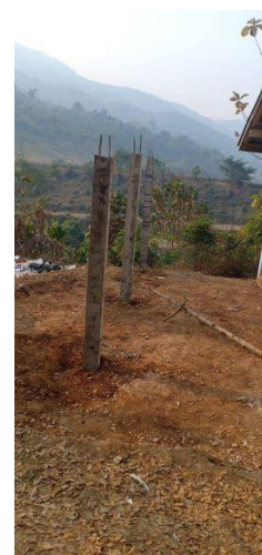
Preparing to build the water trough
